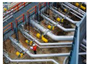
General Pipeline Service
